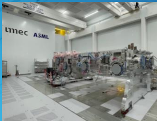
Litho Cluster: track installed, system install started
