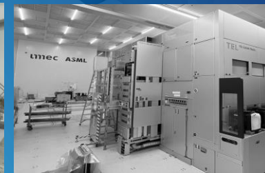
Litho Cluster: track installed, system install started
